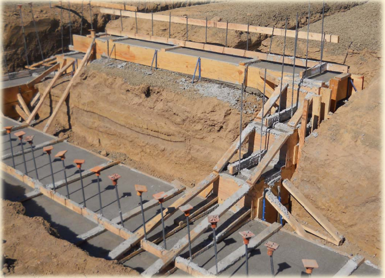
Wet concrete placed into the footing formwork
